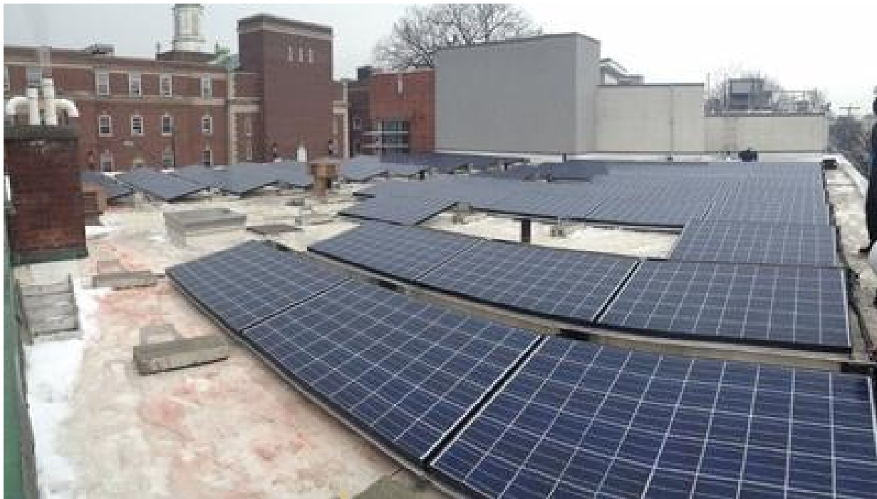
Figure 3: Panels Installed on Our Roof
